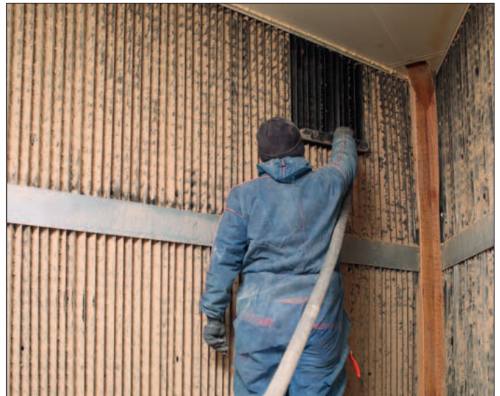
Cleaning the filter with a brush
