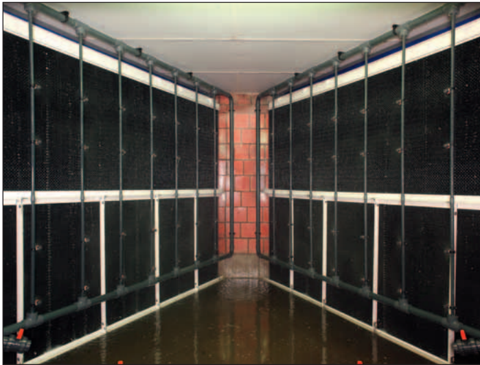
The nozzle group sprays water onto the front of the filter bank
