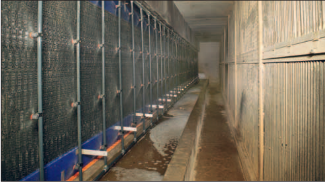
Using MagixX-L in an aviary house for laying hens
