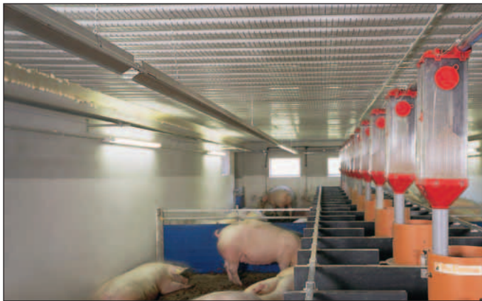
Delta pipe for assembly beneath Diff-Air ceiling
