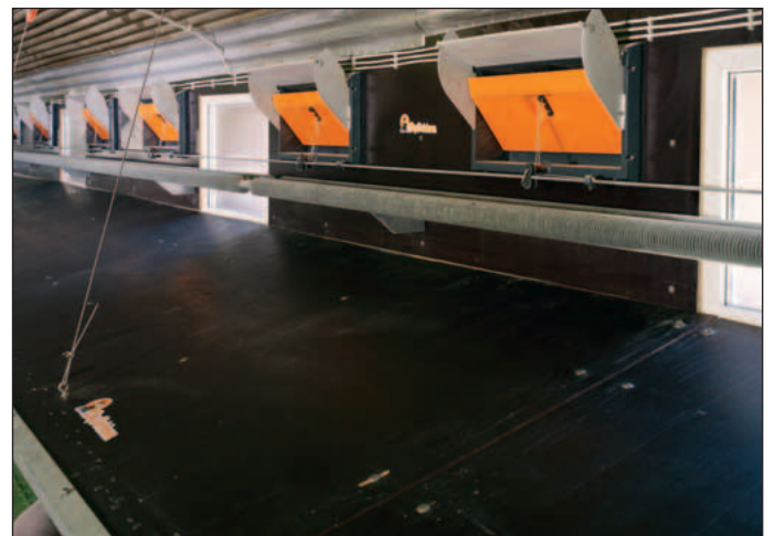
Fin heaters – ideally suited in combination with CL 1200 air inlets
