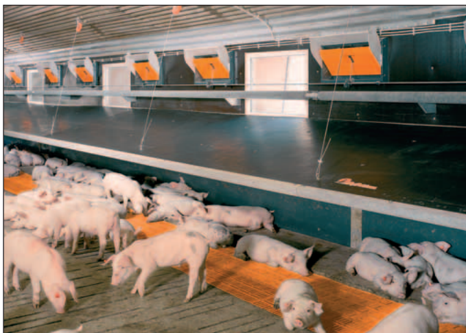
Fin heaters as full-space heating system for piglet rearing houses
