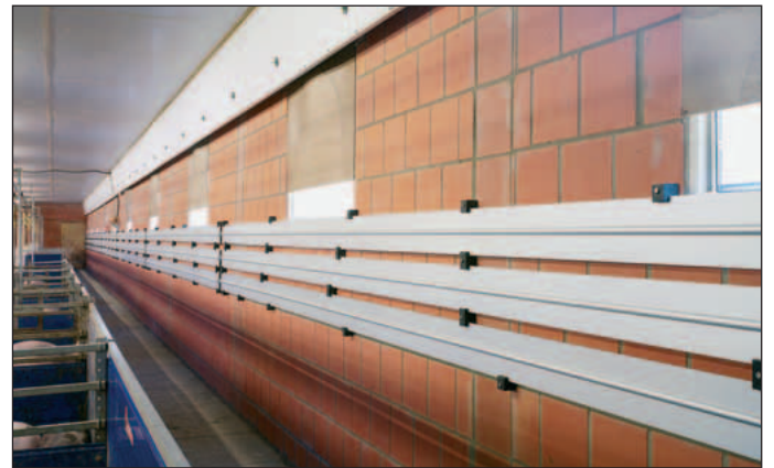
Twin pipe for wall-assembly, less dust on pipes
