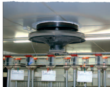
FAC fresh air chimney with protection screen (option) and recirculation unit
