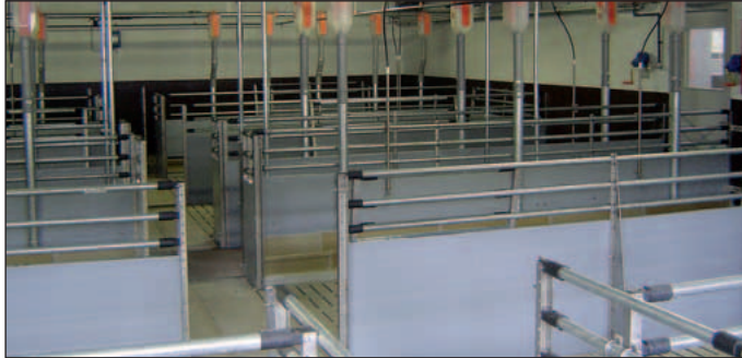
Reinforcing stands installed in the waiting area
